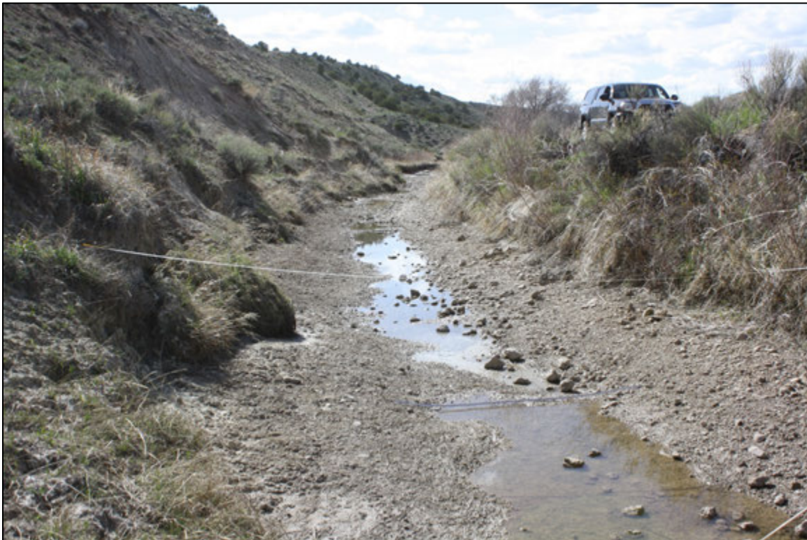
Photo 4. Maybell Canal overview, view to the west.
