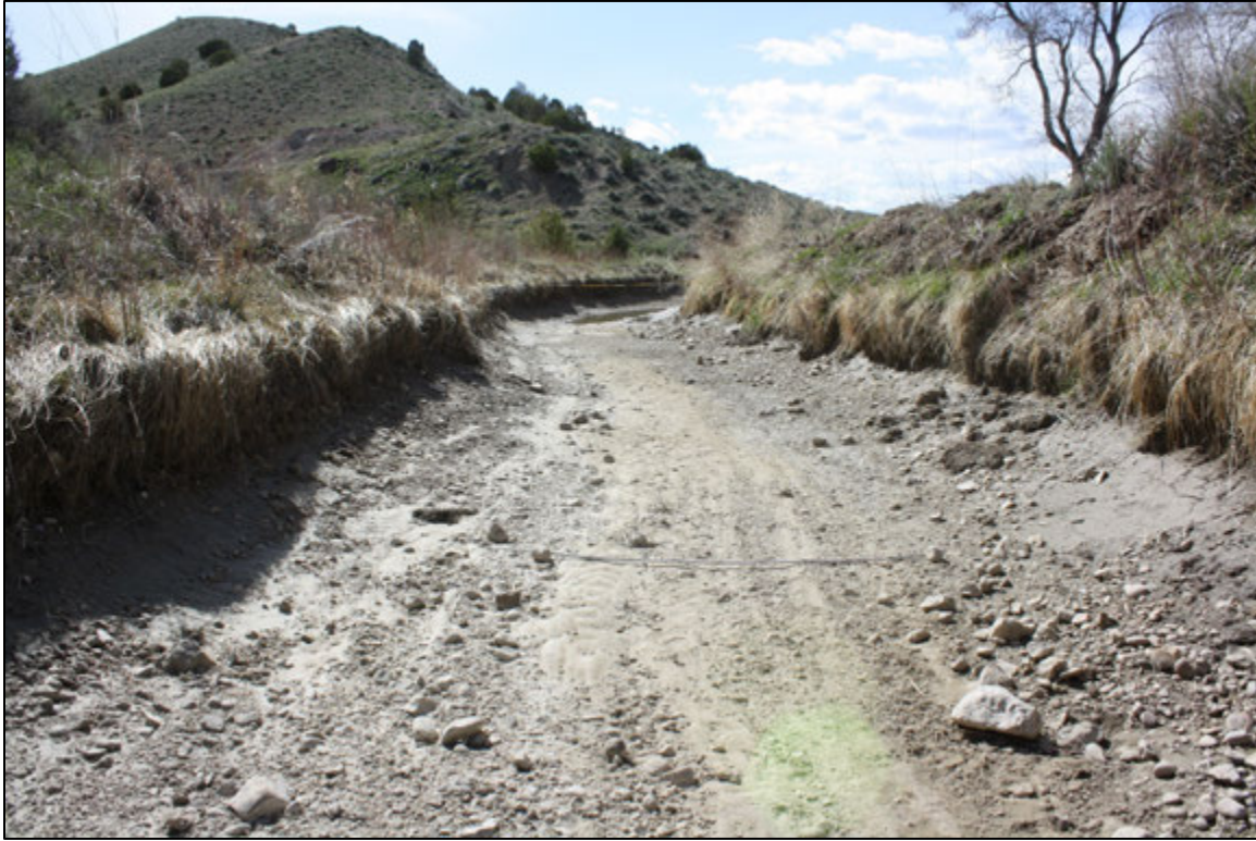
Photo 1. Maybell Canal overview, view to the west.
