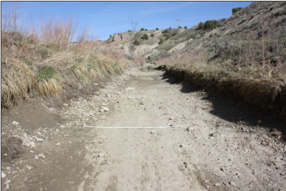
Photo 2. Maybell Canal overview, view to the west.
