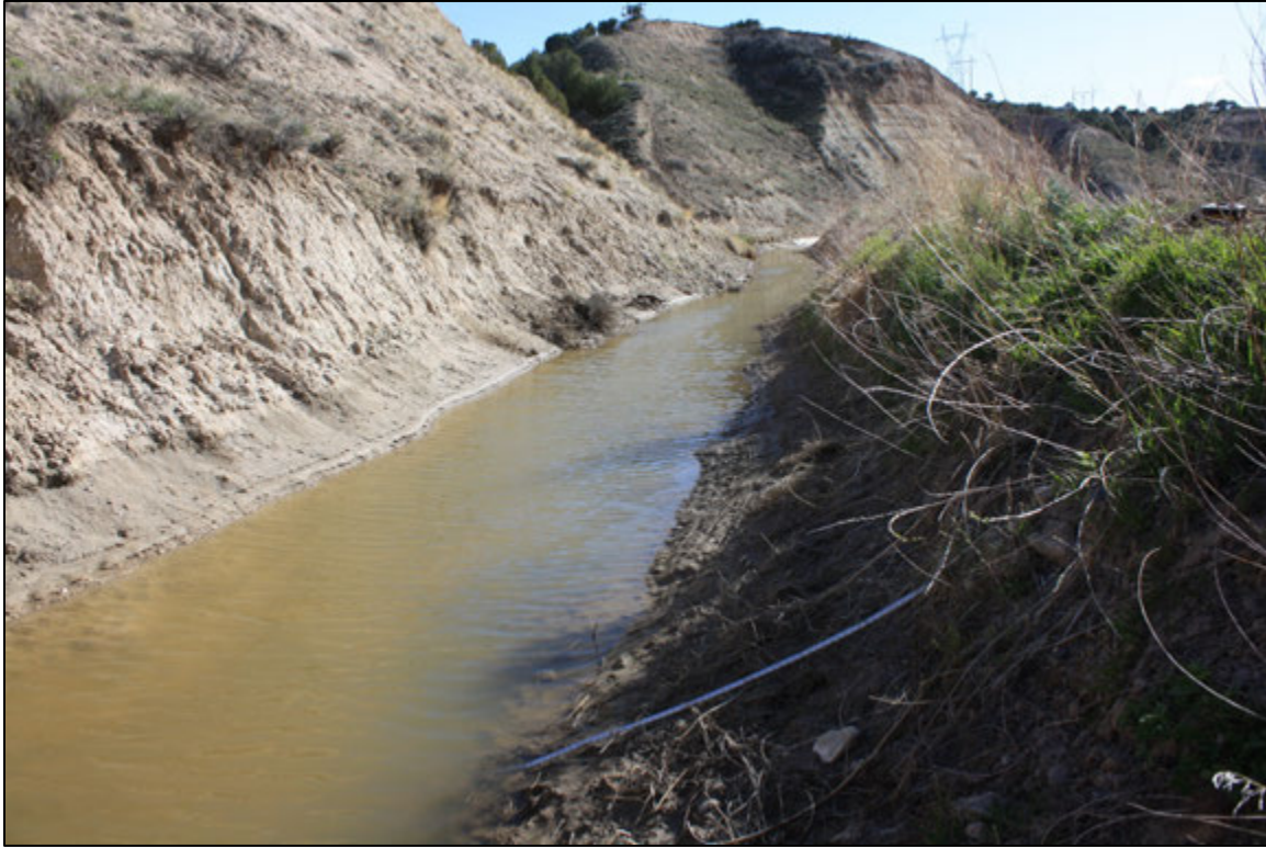
Photo 9. Maybell Canal overview, view to the southwest.
